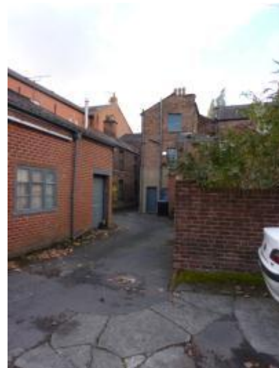
Photograph 25: Rear of Market Street
