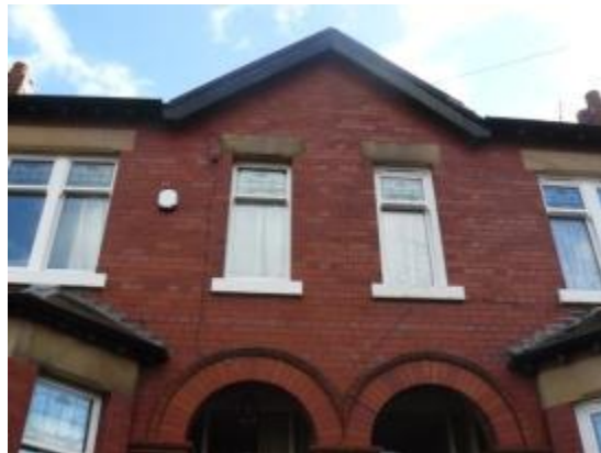
Photograph 77: Timber sash windows with decorative glass
