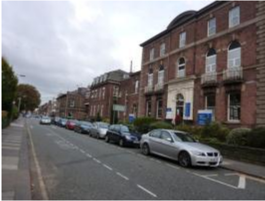
Photograph 34: South End of Market Street
