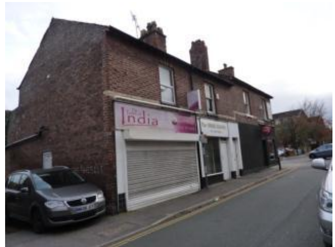
Photograph 88: Inappropriate Signage and Roller Shutters
