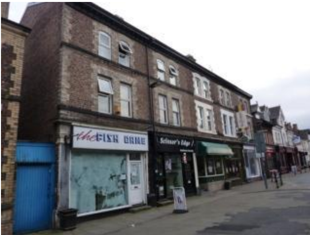
Photograph 87: Vacant Shop Premises with Inappropriate Signage
