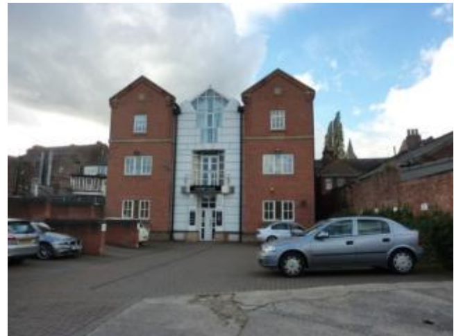
Photograph 96: Area of Cracked Tarmac
