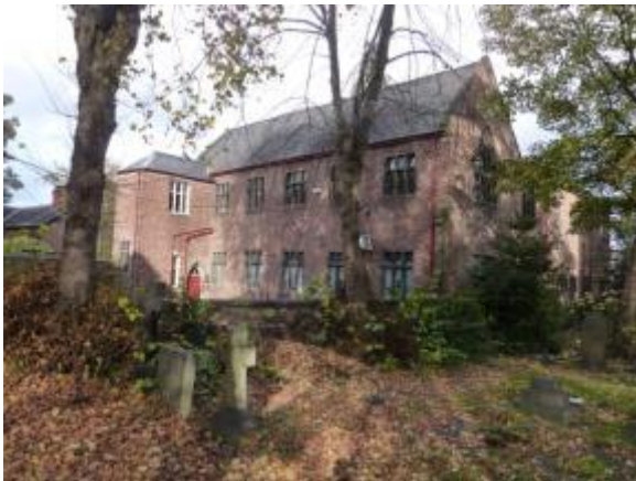
Photograph 17: Undertakers to be included in boundary extension
