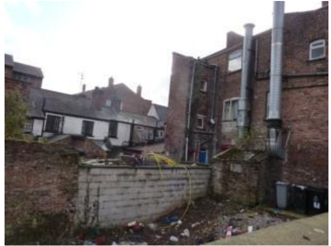
Photograph 85: Inappropriate Ventilation
