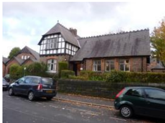
Photograph 69: Former School Building, Sylvan Grove
