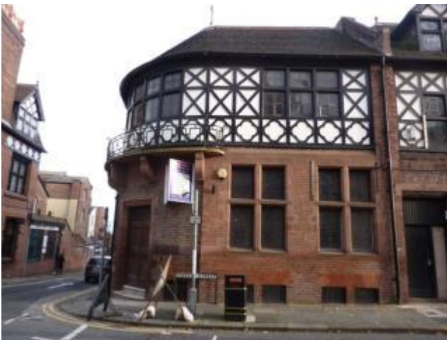
Photograph 82: Number 1 Market Street
