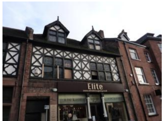
Photograph 83: Number 3 Market Street
