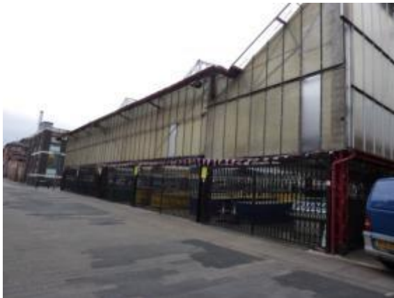
Photograph 45: Side of covered market
