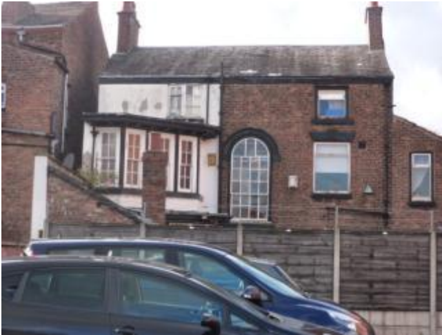
Photograph 84: Rear of Church Street
