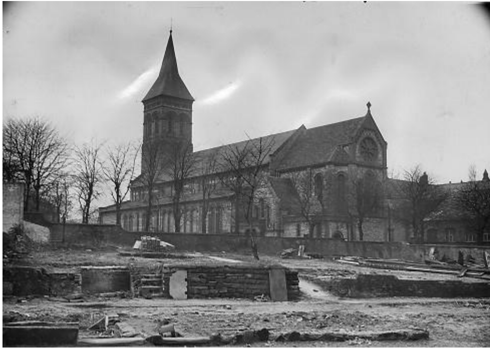
Photograph 5: Demolition in Church Street, 1938 (Trafford Lifetimes, TL3695)
