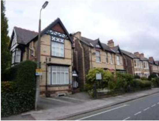
Photograph 62: Residential Properties on Market Street
